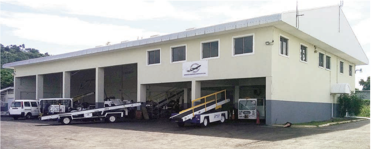
Jamaica Dispatch Services Ltd's new Montego Bay Headquarters in Jamaica.
